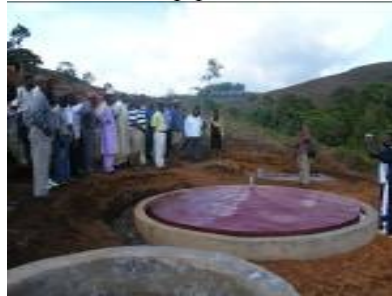
Underground digester with a floating gas holder above.
