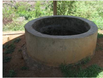
Pre-treatment unit. (mixing chamber) with an inlet pipe.
