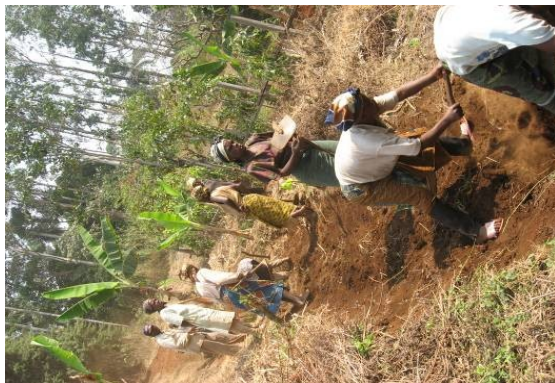
Community participation in digging and backfilling of trenches. plus head load transportation.
