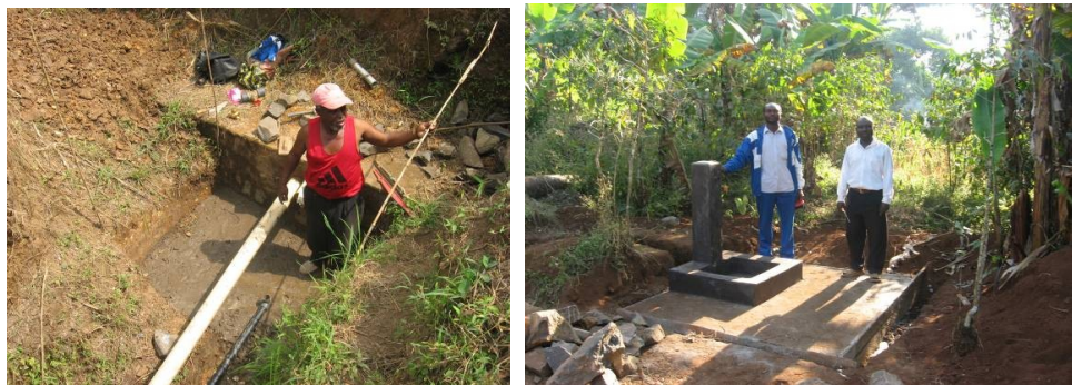
A completed catchmen and satnd tap.
