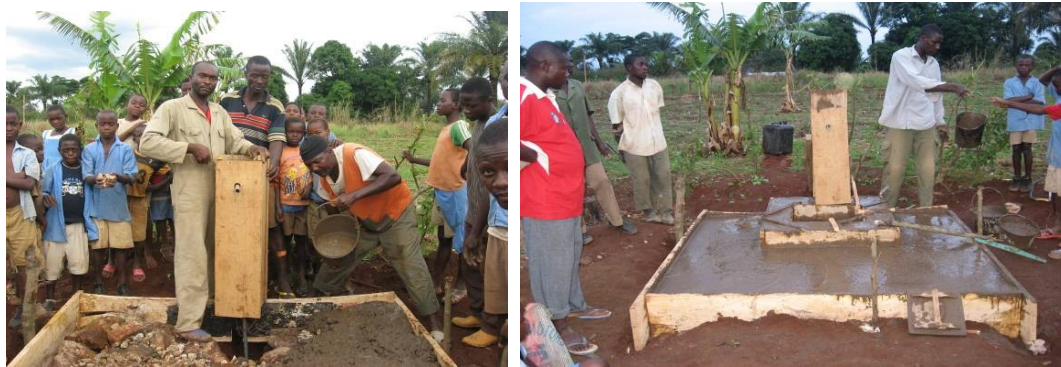
Stand tap under construction.
